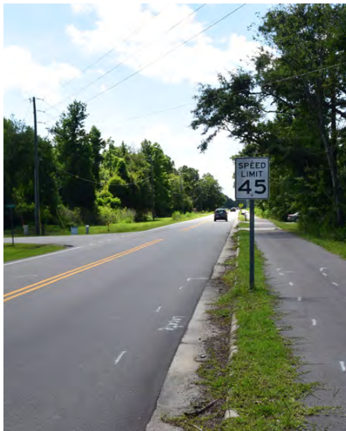
Existing Collector Street, Sloop Point Loop Road
