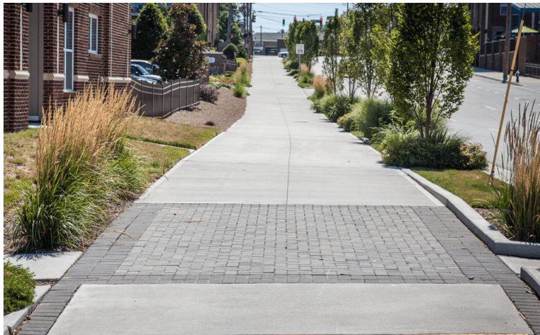
Concrete Trail - Downtown Greenway - Greensboro, NC
