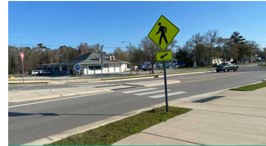
High-Visibility Crossing Over Atkinson Rd
