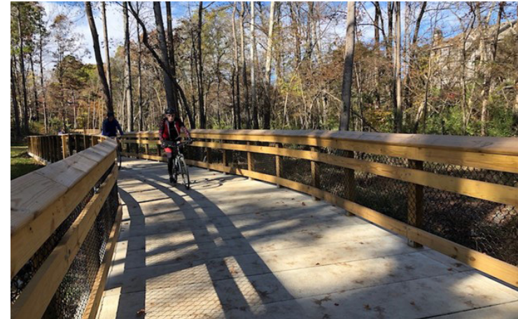
Precast Concrete Deck at Campbell Creek Greenway Ext. - Charlotte, NC Credit: Permatrak.com
