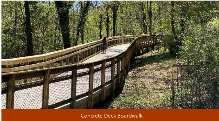
Concrete Deck Boardwalk
