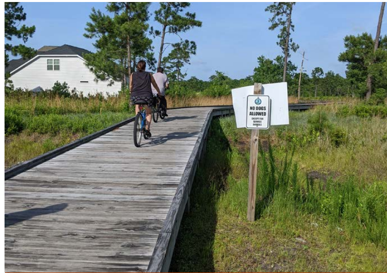
Existing Boardwalk at Hampstead Kiwanis Park - Hampstead, NC
