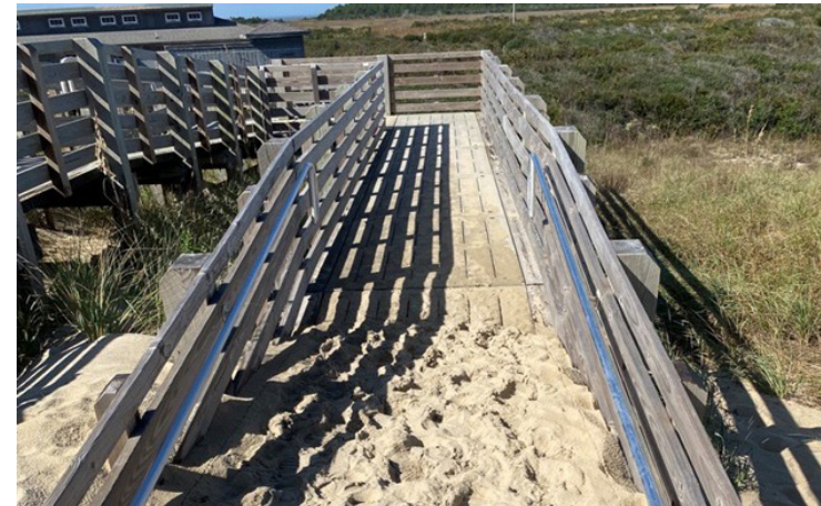
Access Ramp with Slatted Precast Concrete Deck and Sand Accumulation at Coquina Beach - Nags Head, NC
