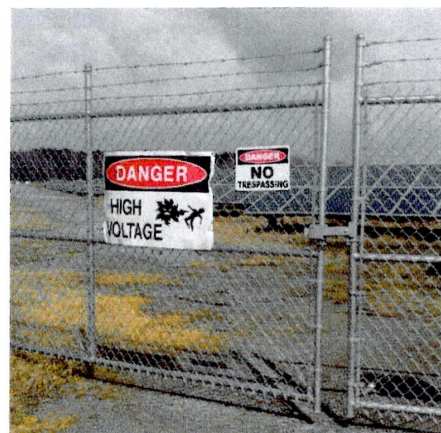
Figure 1. Perimeter Fence with Warning Signs
