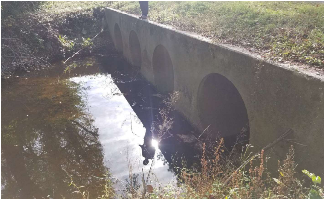
Culvert upstream inlet.
