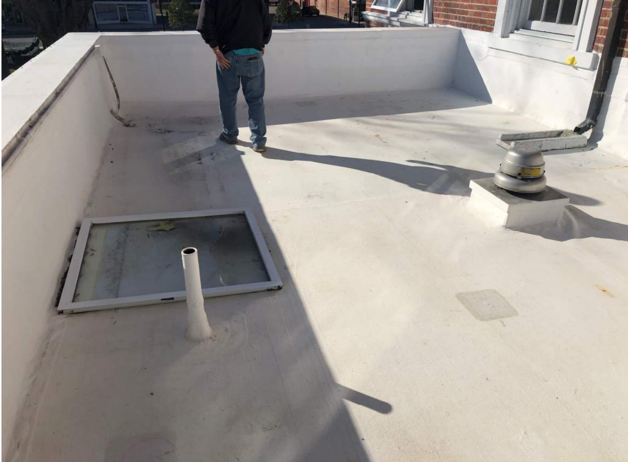
AREA E ROOF (SOUTH FLAT ROOF)
