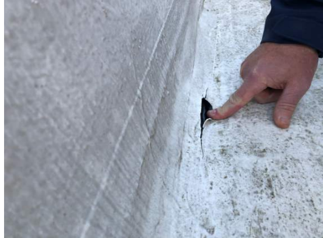
AREA A ROOF (NORTH FLAT ROOF)
