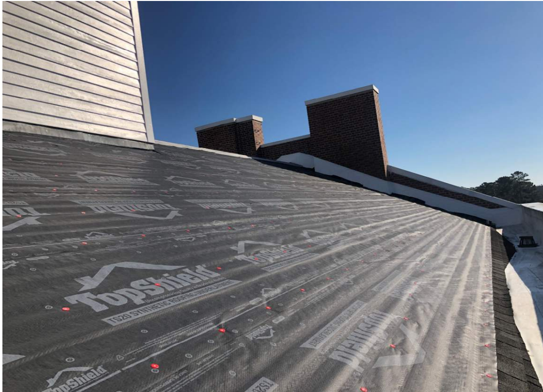
AREA C ROOF AFTER RE-POINTING
