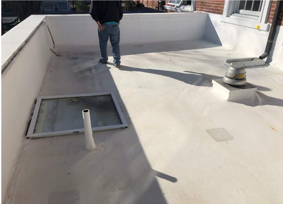
AREA E ROOF (SOUTH FLAT ROOF)
