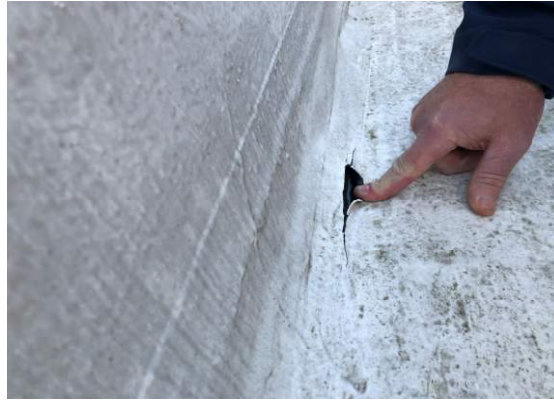
AREA A ROOF (NORTH FLAT ROOF)
